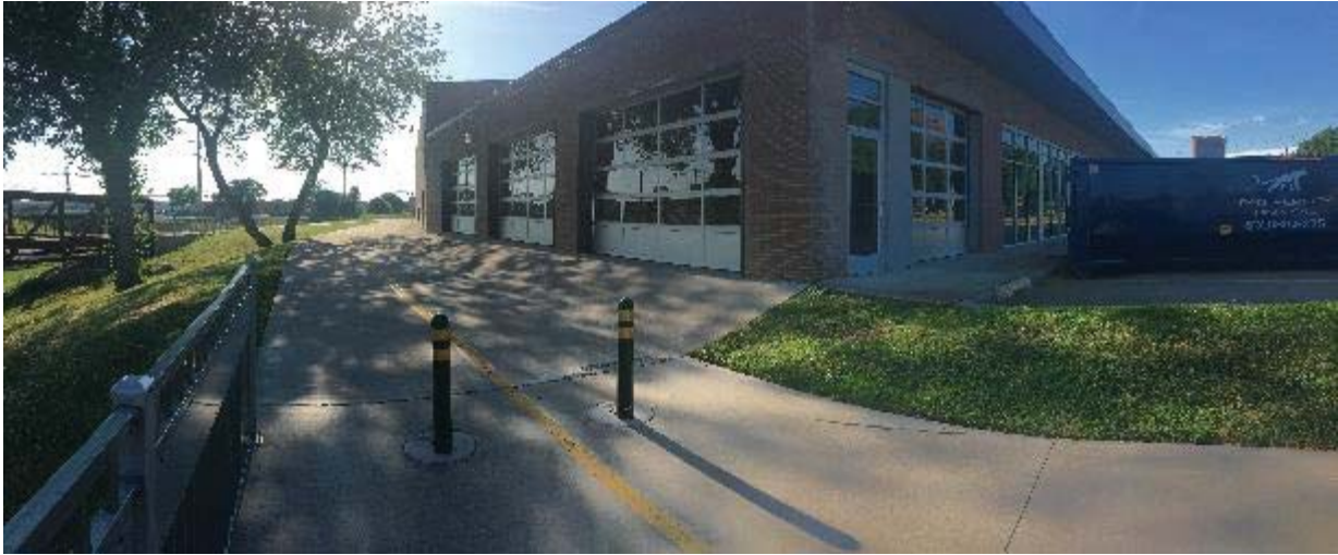
Back of Building #1
